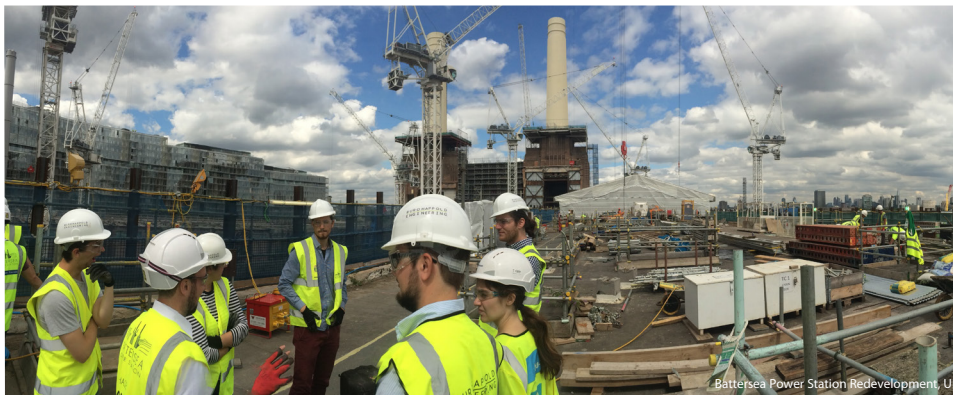
Battersea Power Station Redevelopment, UK
